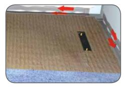
Where the shower tray meets the wall apply a thin layer of Pro-SEAL tape sealer to the shower tray and the adjoining wall approximately 60mm wide on both.
