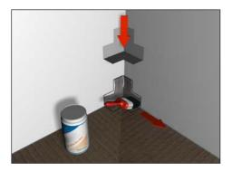
Put on the protective gloves and wear eye and breathing protection. Using the tape sealer and paintbrush, apply a thin layer of tape sealer to the internal corners of the shower area, slightly bigger than the pencil line marked in step 14.
