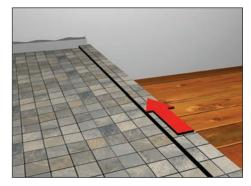
Place the disposable tiling aid into the shower drain hole on the shower tray. The tiling aid provides the edge that needs to be tiled up to whilst protecting the drain from debris. At this stage we recommend fitting tile trim to c eate a clean finished edge for the waste cove.
