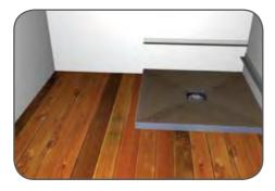
7. You will need to tape all joints where the tray meets the adjoining wall/s. Cut lengths from the roll of Waterproofing Tape and set aside for the moment.
