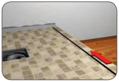
14. After tiling the base of the shower area, we recommend that you add a further narrow border of tiles approximately 30mm to 40mm wide, along the top of the outside edge to act as a water retainer, stopping water running out of the shower area. The tiling aid can now be removed and disposed of.
