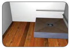
You will need to tape all joints where the tray meets the adjoining wall/s. Cut correct lengths from the roll of Waterproofing Tape and set aside for the moment.
