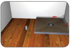
12. Place the strips of Waterproofing Tape previously cut in step 7 along the edges of the shower area, folding half up the wall and half on the shower area as you go. Press firmly into the tape sealer and the tape should also overlap the Waterproofing Internal Corners. When you have finished you can remove the protective gloves and eye and breathing protection.
