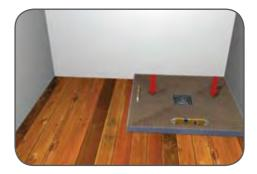
4. Place the Shower Tray into position and bed down onto the adhesive cement. Check that the shower tray is level in both directions using a suitable level.
