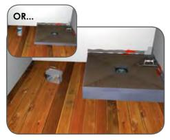
11. Where the shower area meets the wall apply a thin layer of tape sealer to the shower area and the adjoining wall approximately 60mm wide on both.
