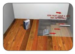
Note: Wear protective gloves, eye and breathing protection. Mix the board fixing adhesive according to manufacturer's instructions to achieve a stiff consistency. Spread the board fixing adhesive onto the floor of the shower position and drag a 6mm notched adhesive trowel across the surface. The notched adhesive trowel will make a ribbed pattern which will leave just the right amount of adhesive on the floor.
