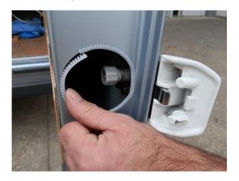
9) Position lock and gasket ensuring gasket arrows are upward. Insert and tighten 8 x socket cap screws complete with washers.
